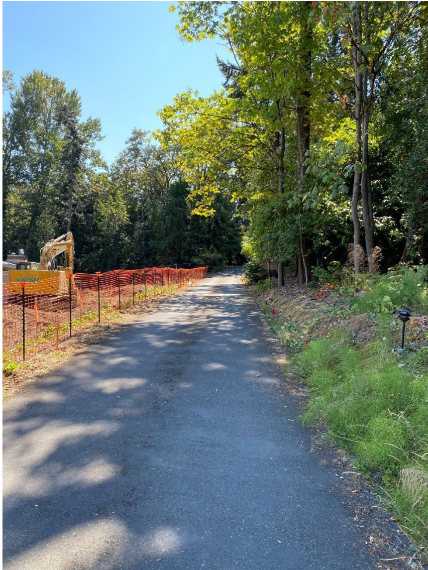
View looking south of existing paved access drive along east property line.
